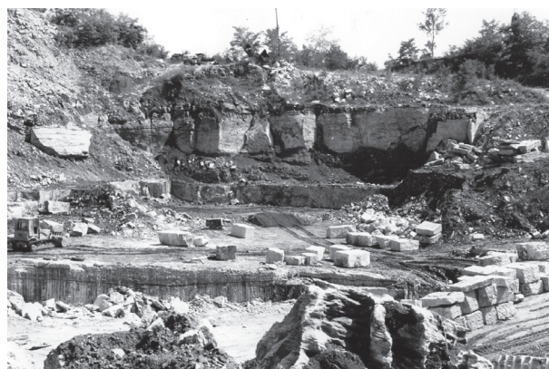
Fig. 3. Cencio dell’Orbo Quarry. From the top to the bottom: a) upper volcanites, b) upper member of the “Chiampo Limestone”, c) volcanites with Lophoranina and sponges, d) lower member of “Chiampo Limestone” (bottom of the quarry).
