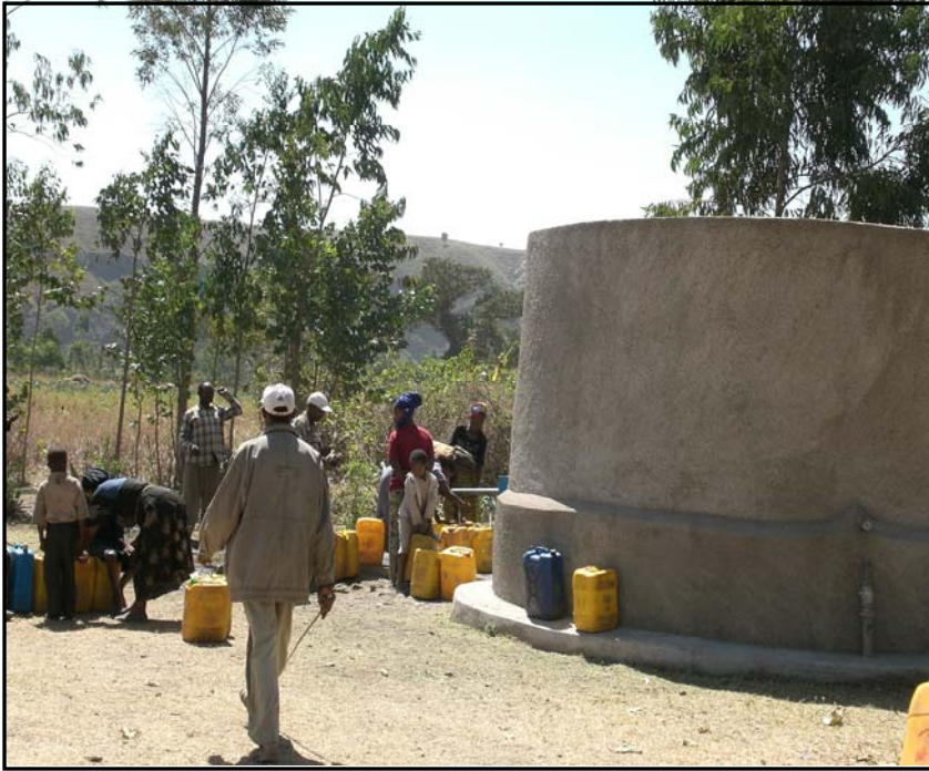
Figure 2.6: Community water supply well from the study area (photo: January 2007)
