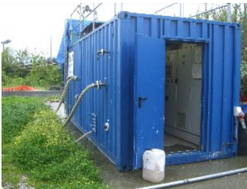
(a) La Spezia MBR pilot plant
