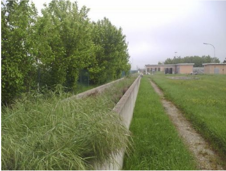
Figure 4.25.: Ferrara H-SSF pilot plant for the first investigation
