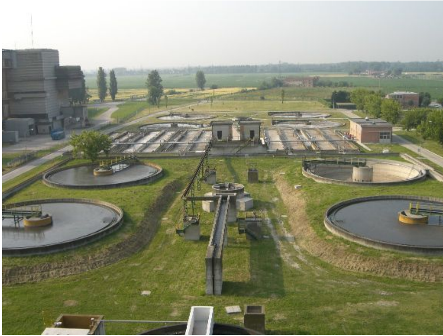
Figure 4.23.: Ferrara WWTP with the two lines for urban and industrial WWs
