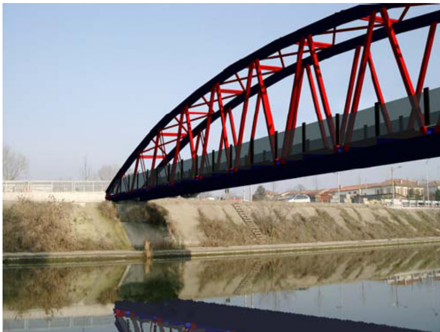
Figure I.2. Proposals for an FRP footbridge across the river Po di Volano in Ferrara (MSc theses by Bruzzo PM and Minghini F, Ferrara University 2004).
