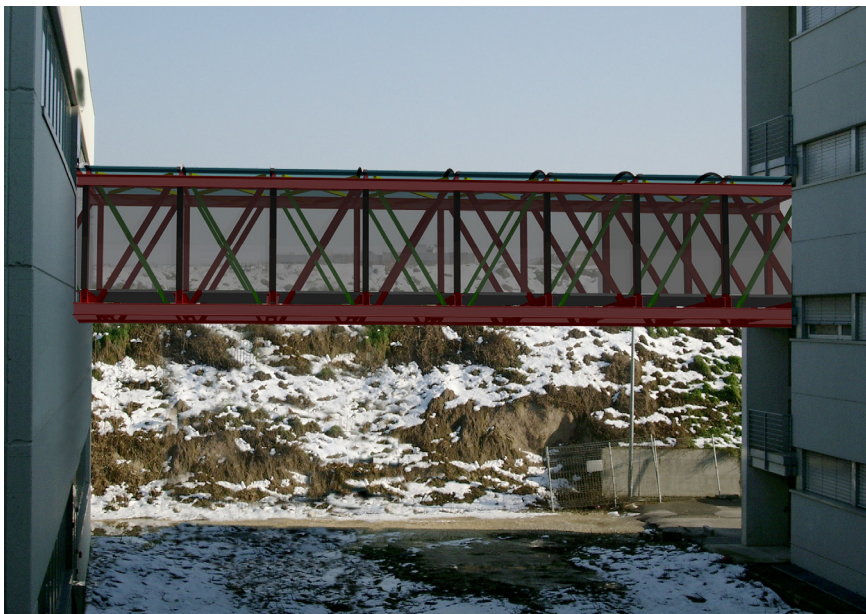
Figure I.1. Proposal for an FRP footbridge connecting two buildings of the Scientific-Technological Pole of Ferrara University (MSc thesis by Bruzzo PM, Ferrara University 2004).
